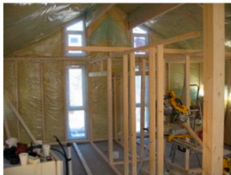
Building structure finished, Inside work on track
