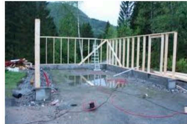
Foundation finished, building structure started
